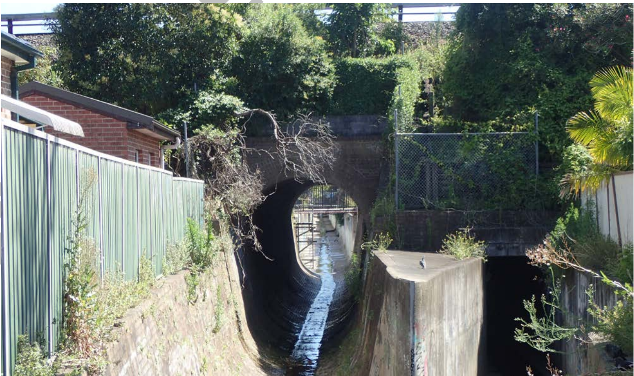
Figure 13: Looking north along Iron Cove Creek at the Western Railway - 1890s oviform channel on the left and culvert on the lower right
