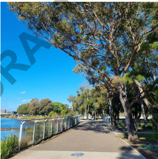
Bridge over side channel at Cahill Park, Wolli Creek
