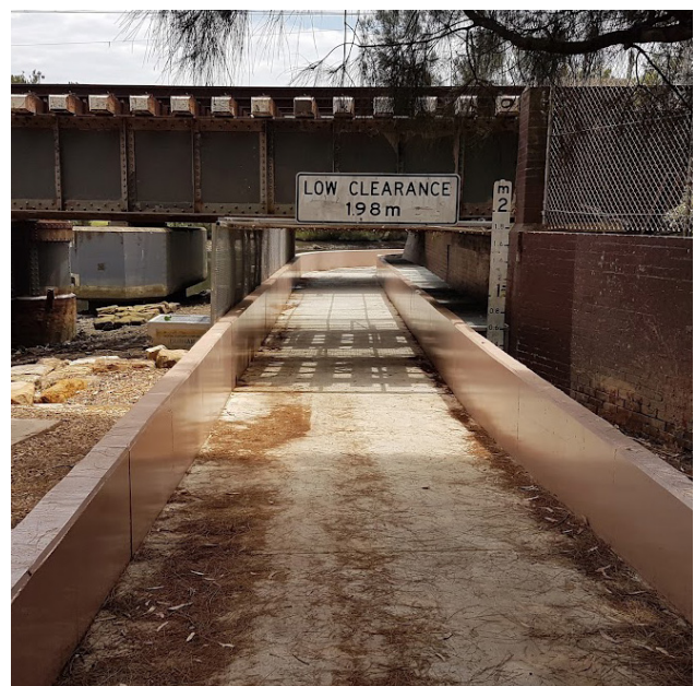
Figure 26: Underpass, Cooks River, Tempe
