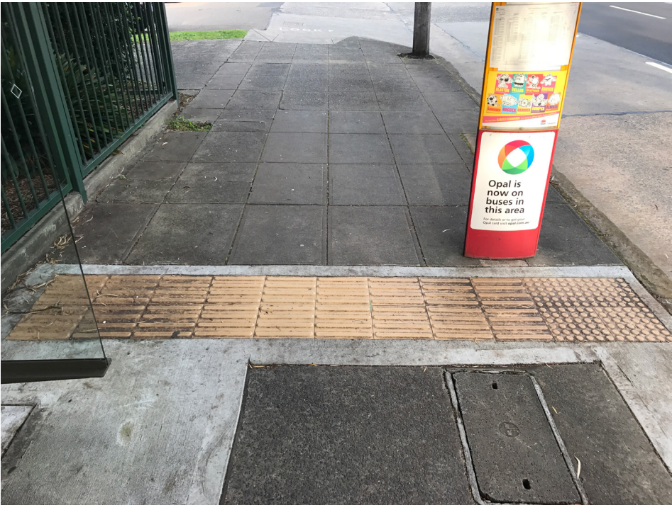
Marrickville Road's north side, existing bus stop. Tactile indicators
