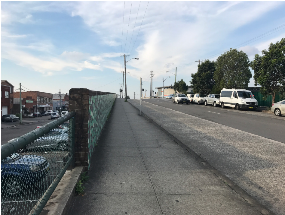
Railway Parade's lower end. Western footpath
