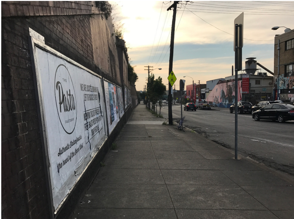
Marrickville Road's south side. Heritage listed retaining brick wall. Looking west
