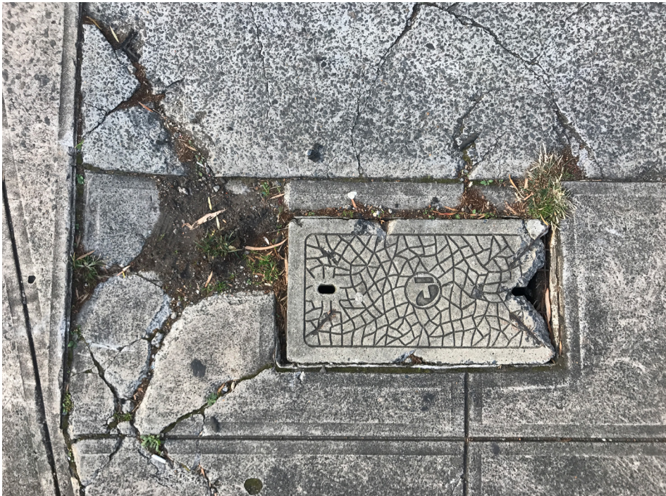
Pavement detail. Marrickville Road, north side.
