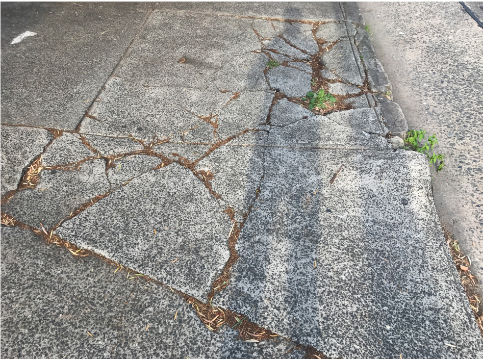
Pavement detail. Marrickville Road, north side., close to Barclay St.
