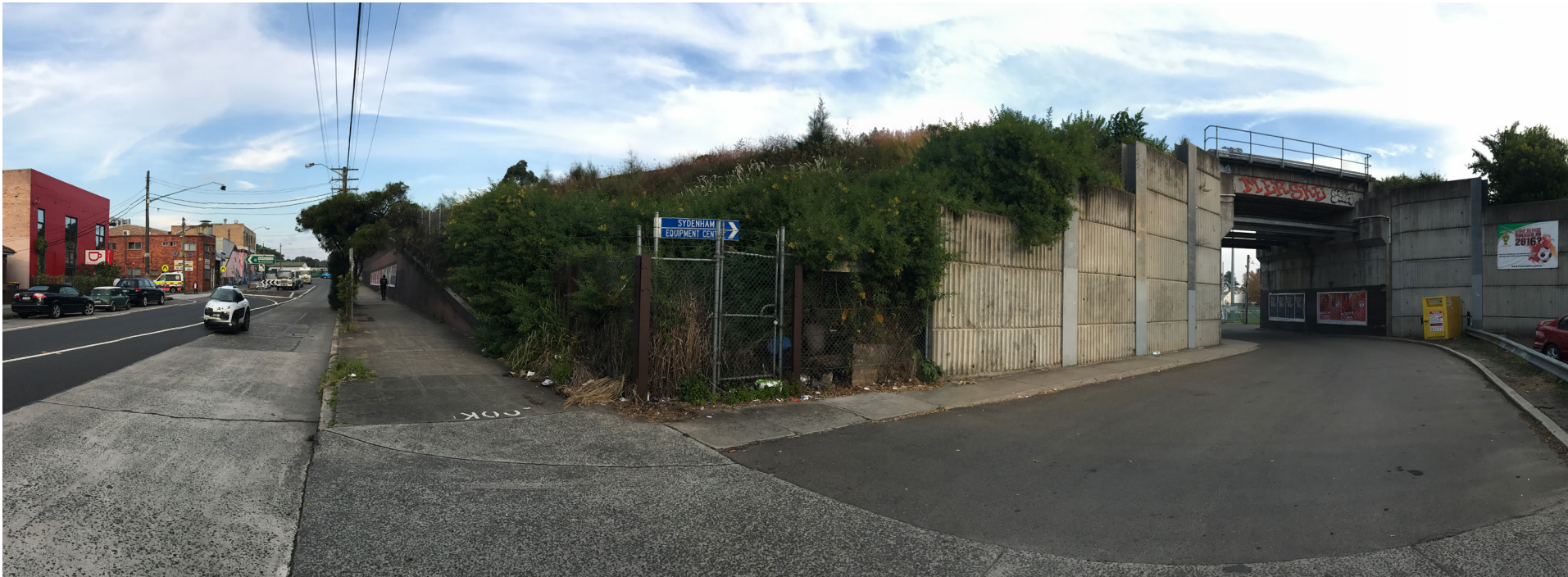
Marrickville Road's south side. Corner with Fraser Park's access lane
