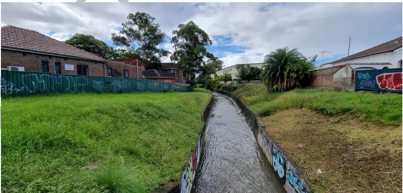
Figure 2: Site photo of an upstream section of the Iron Cove Creek corridor
