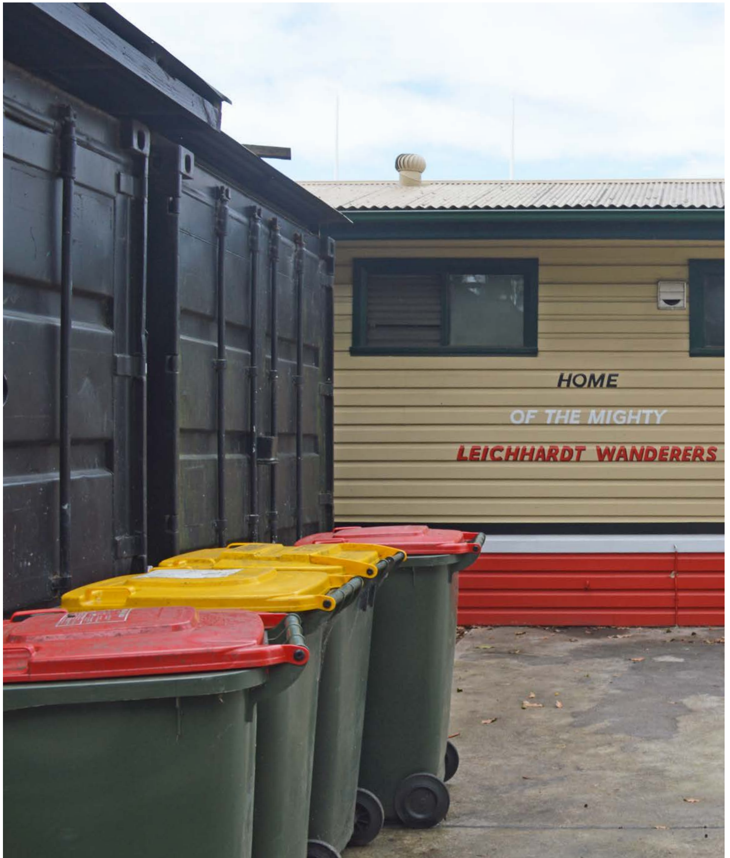
Clubhouse courtyard + Canteen. Photography by Welsh + Major.
