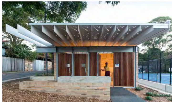
Cohen Park Amenities on Gadigal Land, Annandale Sydney Welsh + Major Architects
