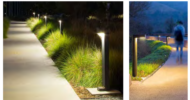
Examples of low level path lighting
