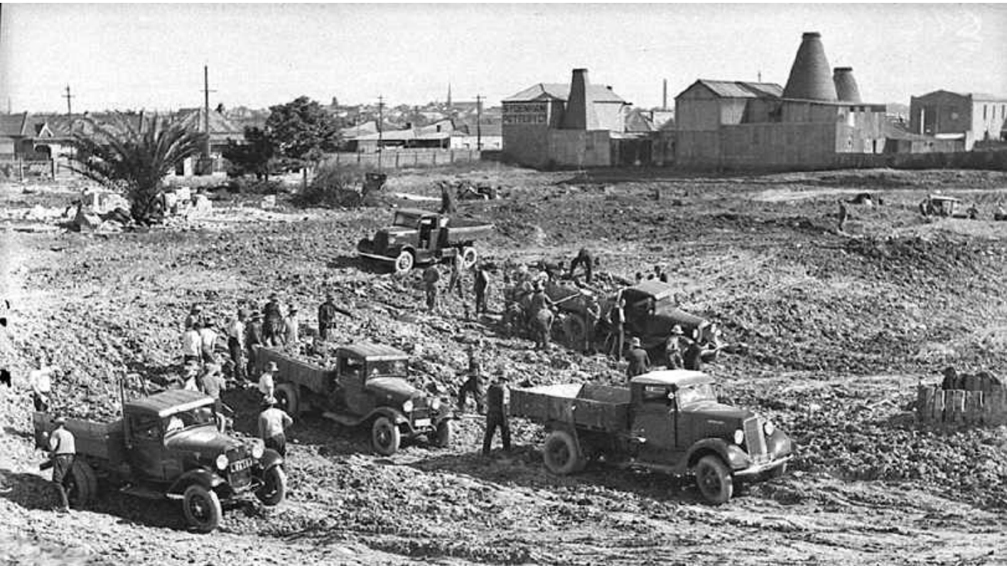
Construction of the stormwater pit in Garden Street Sydenham, 1935. Source: State Library NSW
