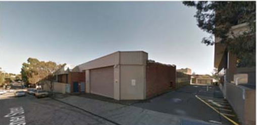
03 VIEW TO SUBJECT SITE FROM FISHER STREET
